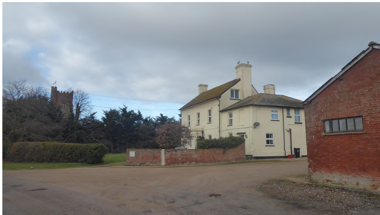
Figure 39 View 10 Holland Hall and the Church Tower looking west
