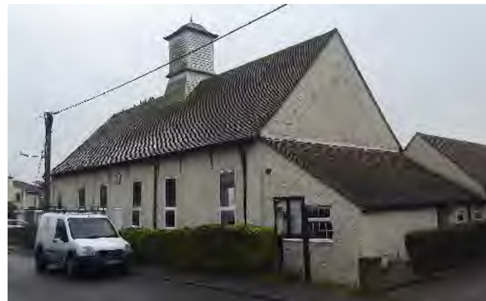
Figure 27 The Village Hall Manor Road
